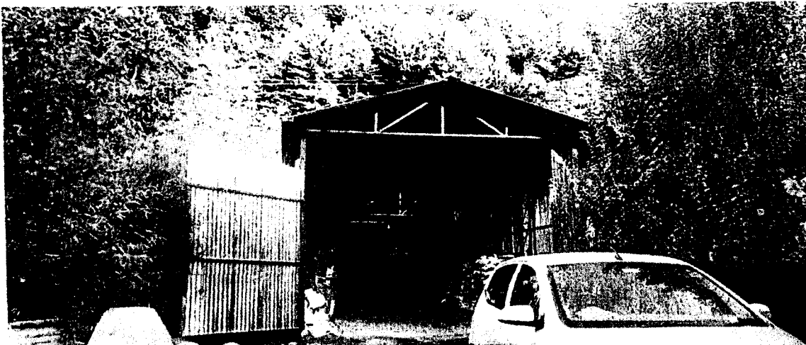
Fig: Entrance of MRF site of M/s Krich Cleaning Pvt. Ltd. Village Mansari, Distt. Kullu.
